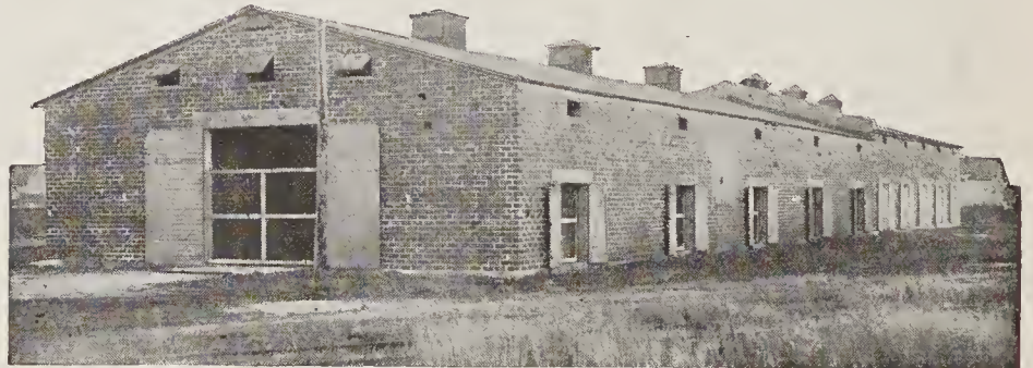
One of our 8 Frost-proof Onion Set Storage Warehouses, capacity 42,000 bu.
